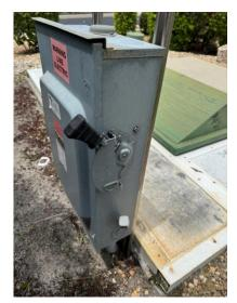
The first and easiest option is to turn off the power at the external breaker by the entrance to the underground vault. This effectively shuts off all power in the vault including a "sump pump" and the various timers which control the pumps and external lighting.
