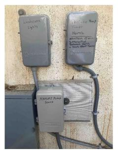
There are three timers. One controls the external fountain area lighting and the other two control the pumps. The timer for the lighting is an intelligent device that uses a combination of WIFI and GPS to turn/off the lights. Nothing needs to be done.
