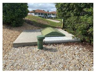
This procedure will include going down into the underground vault where all of the fountain equipment is located. The advantage of this process is that only the two 15 hp pump breakers will be shut off. The timers and sump pump will not be impacted. However, in an elongated power outage, the timers will need to be reset. The green cover must be raised and then you climb down into the vault.
